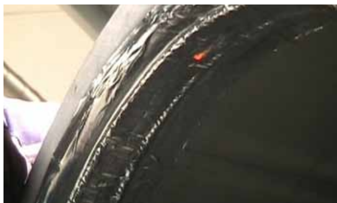
Step 2: Weld onto the Argweld® Purge Tape™
